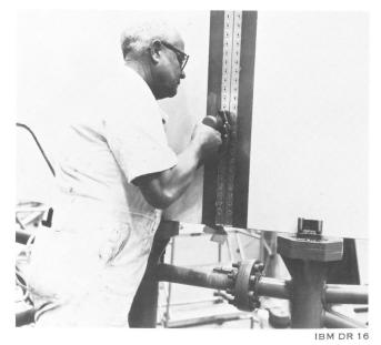
Splice Joint Operations — Final grinding of a splice joint ensures a smooth surface prior to splice plate assembly.
